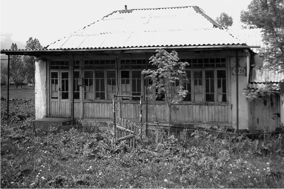
Photograph 25. A house in the village of Dzunashogh (Kyzyl-Shafag), Armenia, 2006. Photo by A. Hakobyan.
